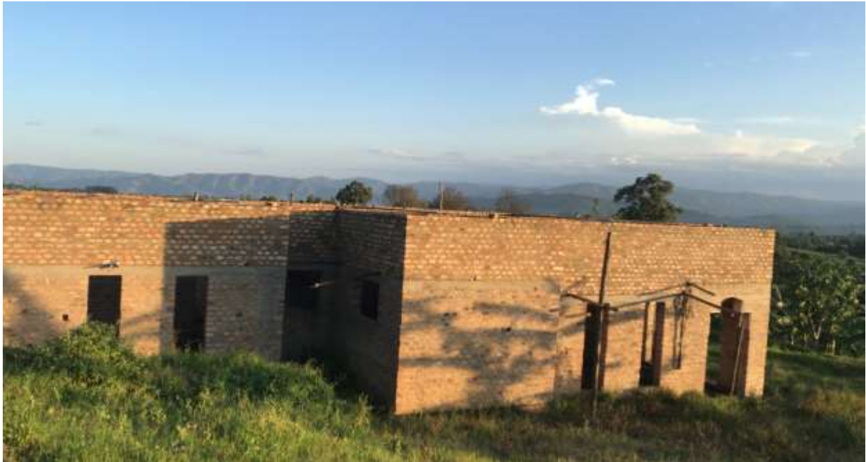
Photograph 2: Family House under construction
